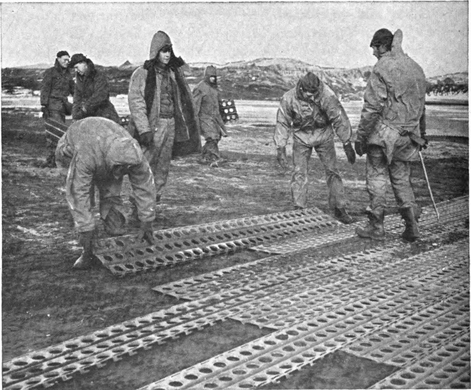
Figure 91. Laying pierced-plank panels. Reversed direction of bayonet hooks can be seen.
